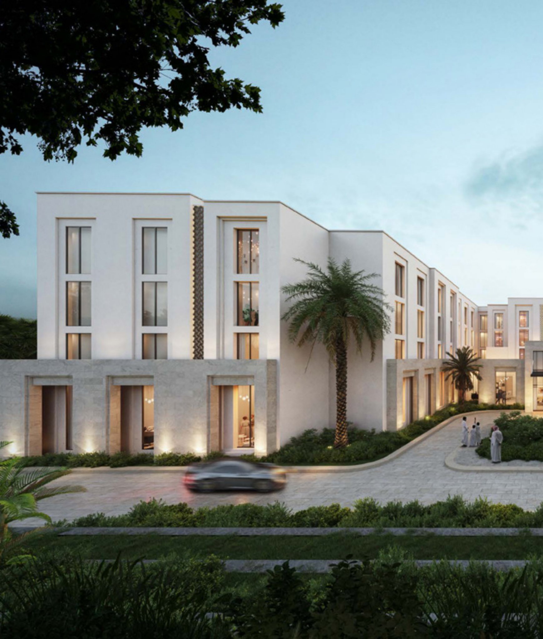
Serviced Apartments Block
